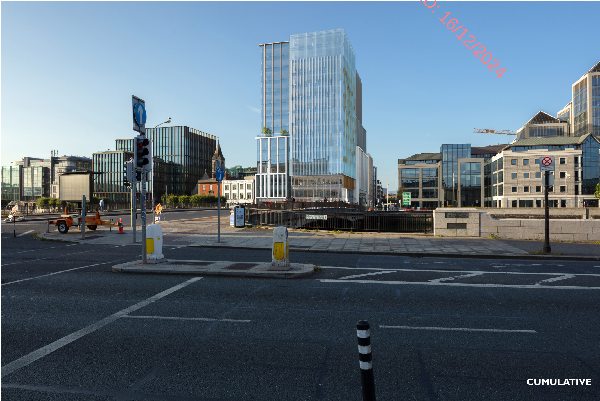
5. Townsend Street / Shaw Street
