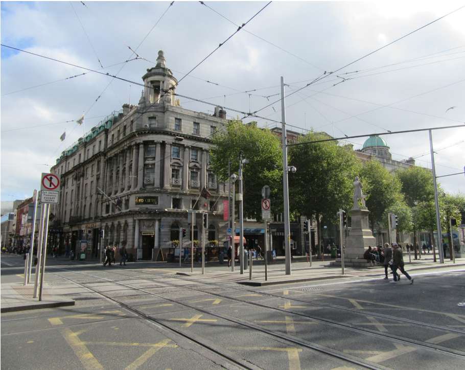
Fig. 9.33: Nos.1-11 O’Connell Street Lower at junction with Abbey St Lower (buildings 6b of this group).
