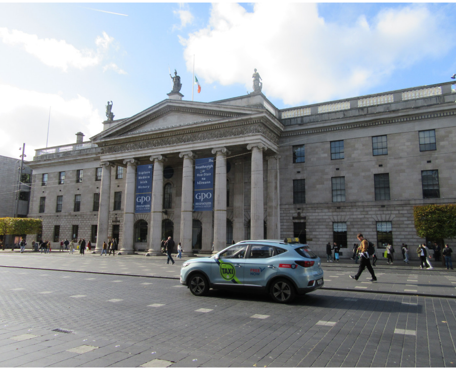
Fig. 9.9: General Post Office (GPO), O'Connell Street.
