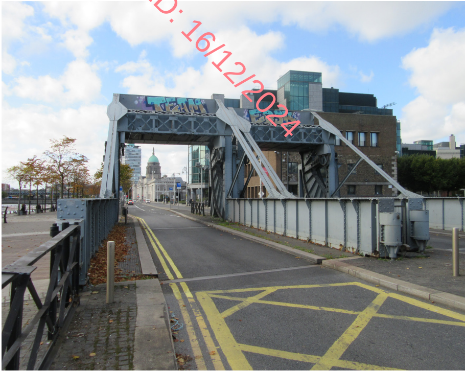
Fig. 9.18: Custom House Quay Bridge, structure 3b of this group.
