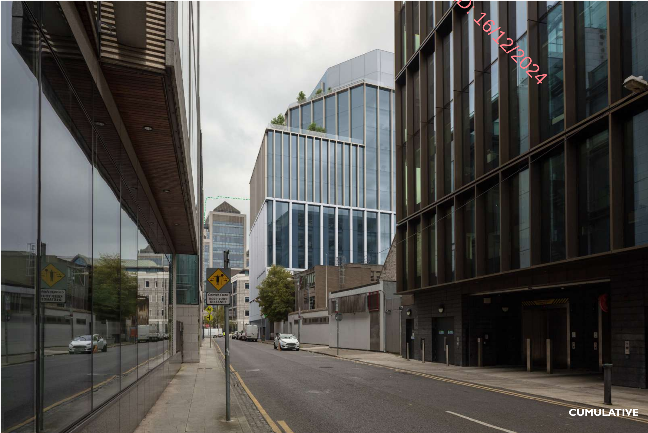
4. Tara Street Tower
