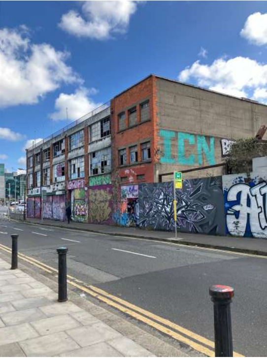
Fig. 4.9: View from Moss Street looking north at the western side of the site.
