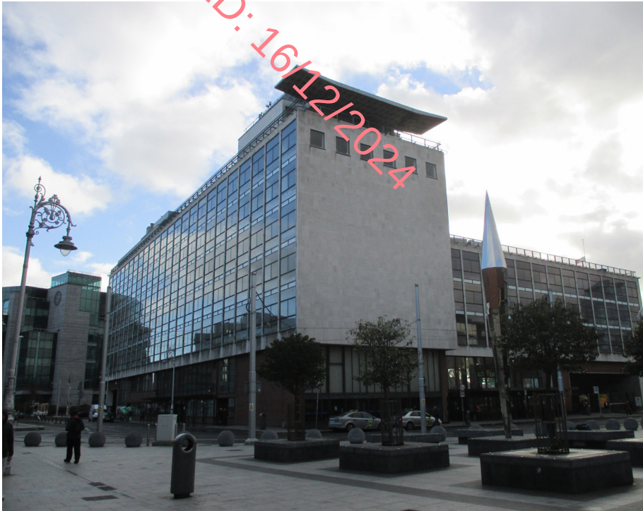
Fig. 9.25: Busáras Station, rear elevation (building 4c of this group).
