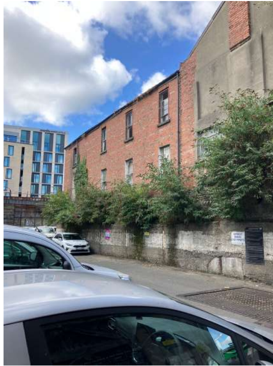
Fig. 4.10: View of the eastern side of the existing building from within the car park area of the site.
