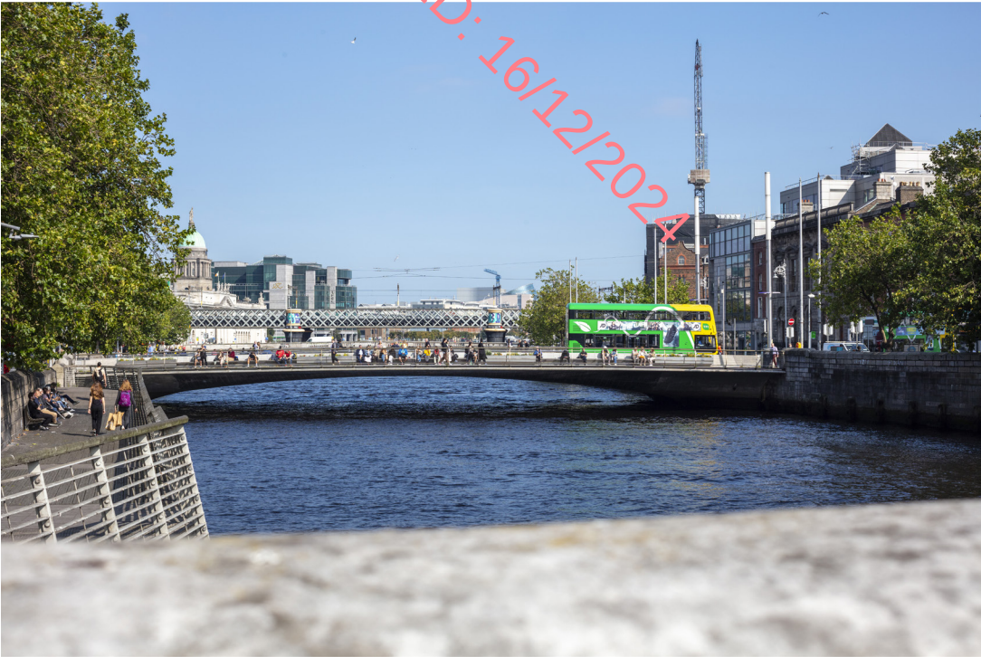
Fig. 9.12: View from the northside of O'Connell Bridge looking east with the Rosie Hackett Bridge in the middle ground.
