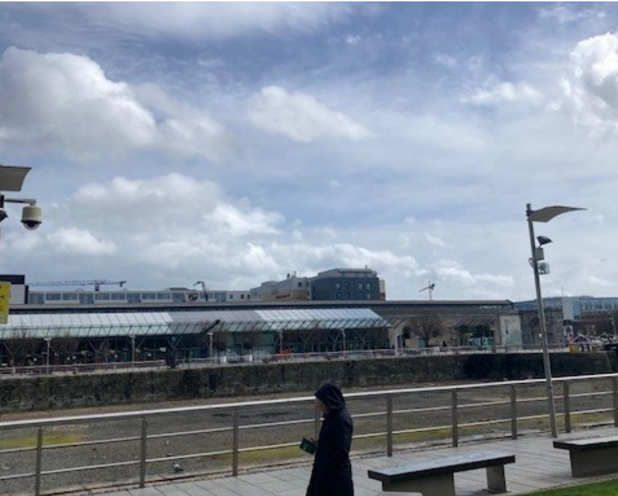
Fig. 9.19: George's Dock, structure 3c of this group.
