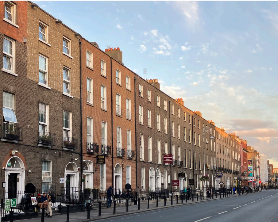
Fig. 9.29: Nos. 71-90 Gardiner Street Lower (buildings 5d of this group).
