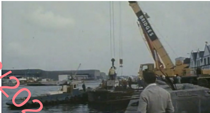
Fig. 3.25: 1977 still from Talbot Memorial Bridge construction - site just out of view on extreme right (RTE').
