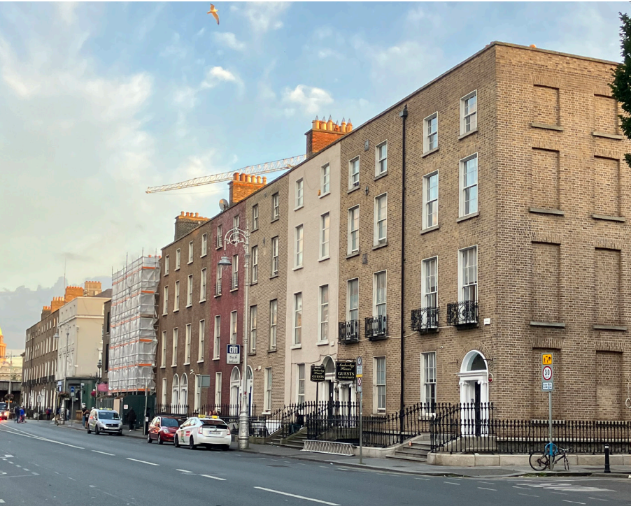
Fig. 9.28: Nos. 33-42 Gardiner Street Lower (buildings 5c of this group).
