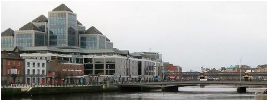
Fig. 3.26: 2018 photograph of the Talbot Memorial Bridge on the right, with the former Ulster Bank HQ on the left and the site below left (Geograph.ie Eric Jones).
