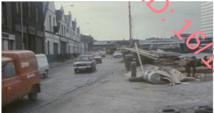
Fig. 3.24: 1977 still from film of the start of construction of the Talbot Memorial Bridge, site is on left just before railway bridge (RTE').
