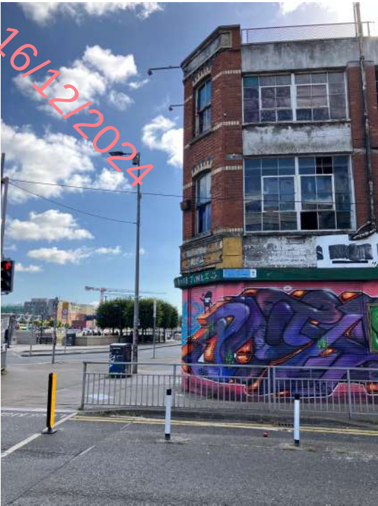
Fig. 4.8: View of the northwestern corner of the site.
