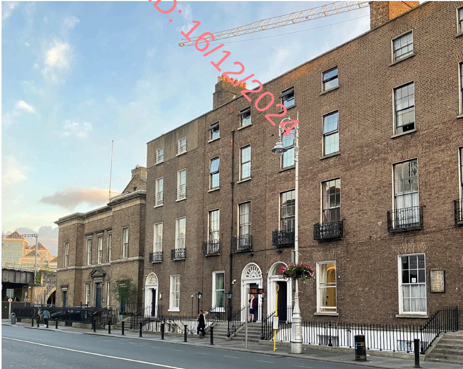
Fig. 9.27: Nos. 43-50 Gardiner Street Lower (buildings 5b of this group).
